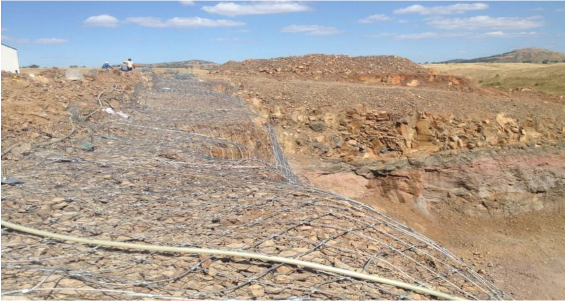
Picture:02 Top Anchoring
